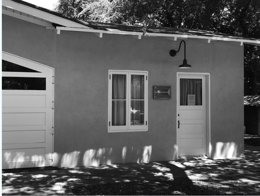
Membership dollars help support on-going preservation work to the Lanterman House, including the repair and repainting of the Visitor and History Center in 2020.
