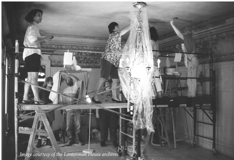
A team of volunteers, under the direction of painting restoration experts Ed Pinson and Debra Ware, carefully clean the ceiling of the dining room.
